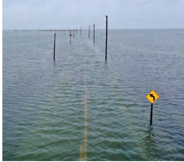
Flooded roads following a nor'easter in Tuckerton, NJ. Photo by Life on the Edge Drones.
