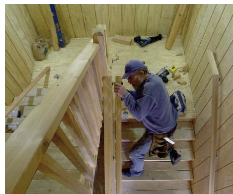
Building a new stairwell. © Jim Briggs
