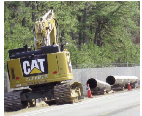
Staging materials along Route 539.
