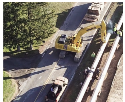
Aerial image of construction along Fisher Road in Plumsted Township.
