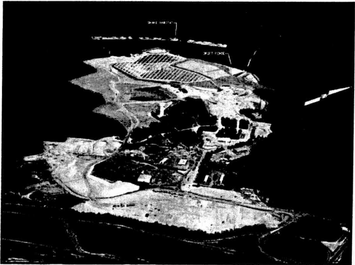
Figure 1. A 2007 aerial photograph showing a western view of the study site and the early stages of the commercial construction on the eastern and central portions of the site. The licenced landfill is centered on the western portion of the SPR property (highlighted with white lines), Retention Basin D is located at the extreme west of the site (highlighted in white), the three pine snake mitigation and management fields are due west of the site (outlined in red lines), and the perimeter exclusion drift fence that surrounds the SPR property (is also outlined with red lines). Source: Walters, Inc.
