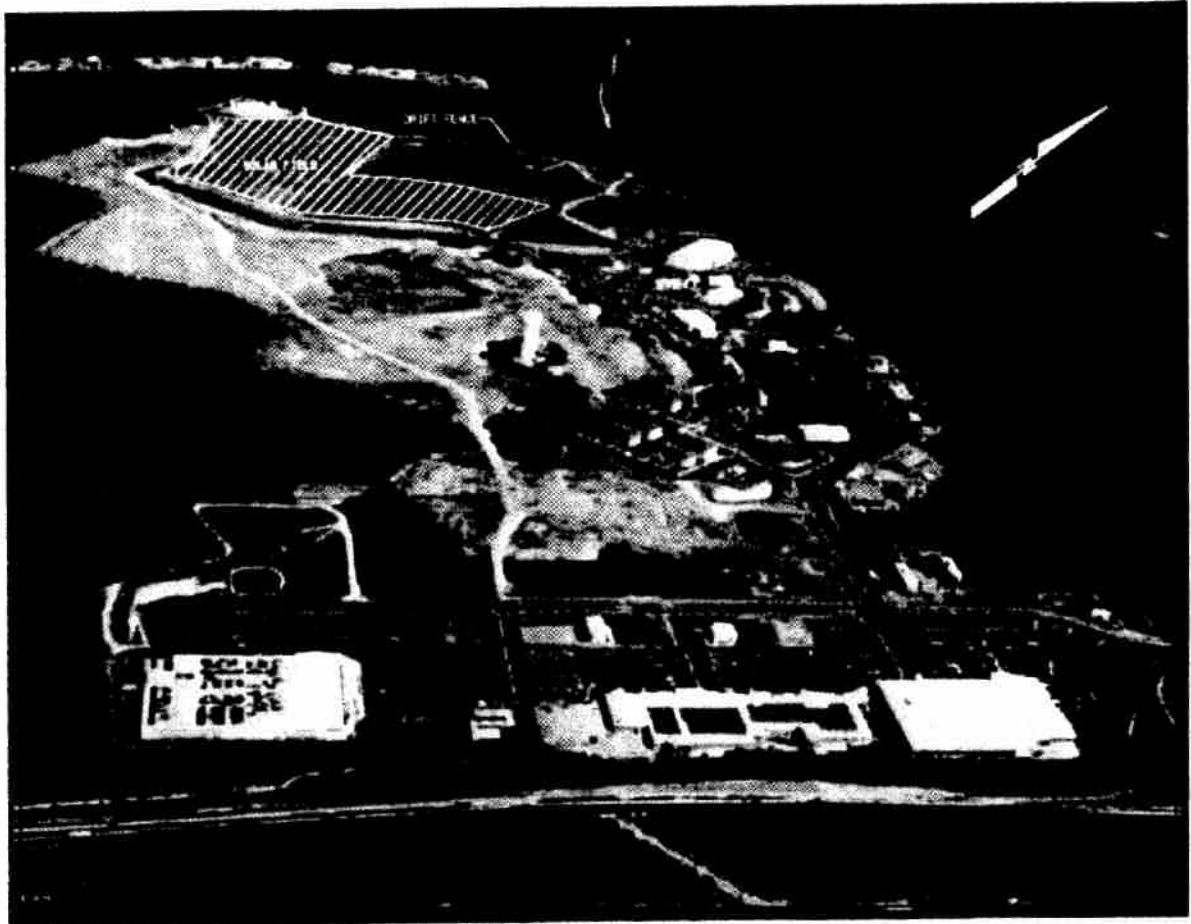
Figure 2. A 2010 aerial photograph showing the approximate locations of the proposed solar panel area on the licensed landfill (the area highlighted with white lines), Retention Basin D (the white area at the extreme top of the photo), the perimeter exclusion drift fence (shown by the red line around the edge of the property), and the existing commercial and residential development areas. The Garden State Parkway can be seen along the bottom of the picture. Source: Walters, Inc.
