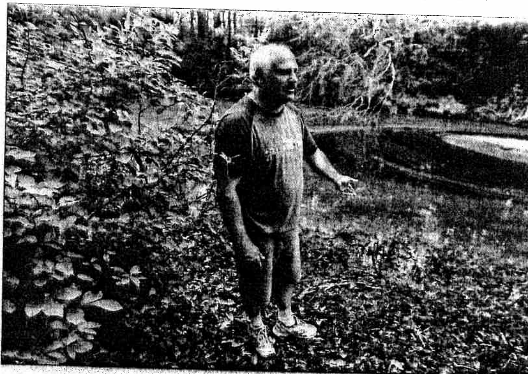
Rich Eggert of Plumsted points to a pond formed by recent rains at a site where the Plumsted Municipal Utilities Authority wants to build a sewage-treatment facility. STAFF PHOTO: BRADLEY J. PENNER
