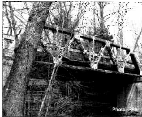
Weymouth Road Bridge
