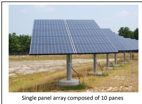
The panel panes are attached in a surface that is closely spaced but not solid. A narrow (~1 inch) space exists between each pane, providing a narrow gap capable of allowing a sliver of sunlight to be transmitted to the underlying shaded area. Each panel is separated horizontally from the
