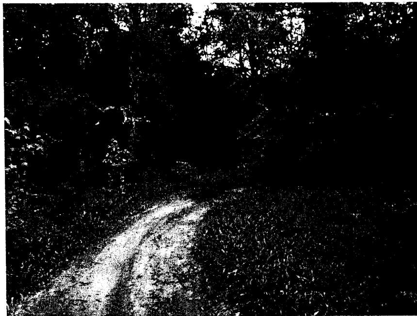
12. Representative photograph of the existing dirt roads that traverse the overall site within the upland areas.
